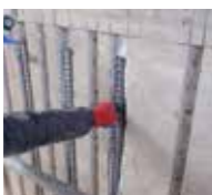
③主鉄筋取付
