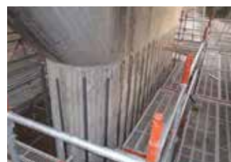
③主鉄筋取付
