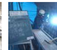
⑤帯鉄筋取付
